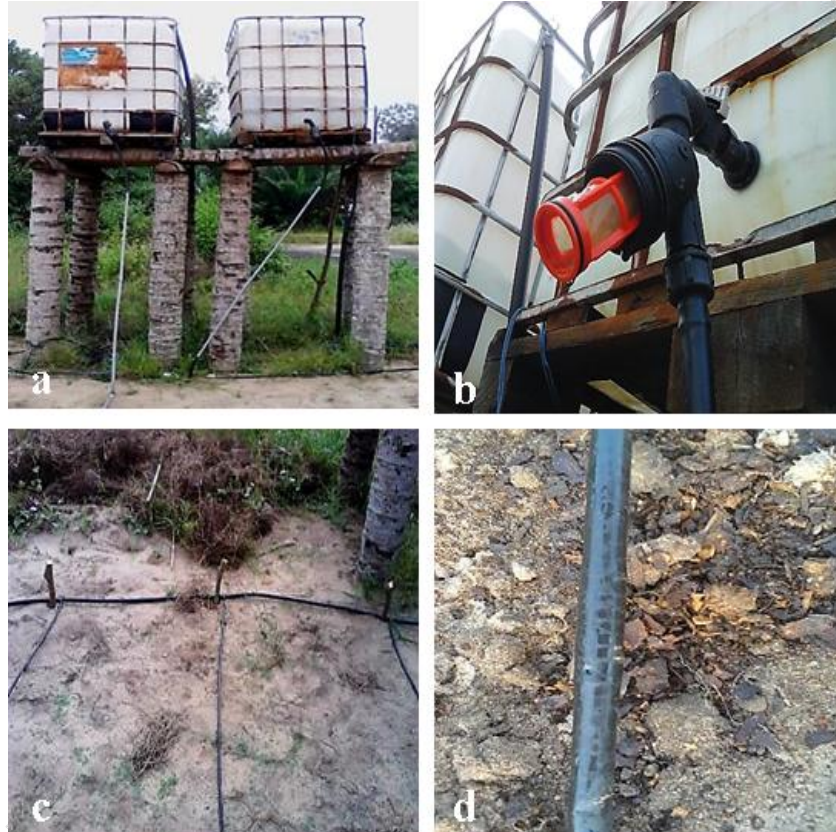
Figure 4. Drip irrigation system consisting of (a) tanks of 1000 l, mounted on supports made of coconut stems 2 m high, (b) filter, (c) ramps and (d) drippers on a ramp.
