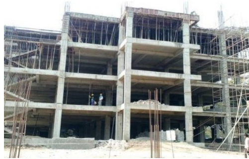
Plate 1. Typical RC frame building [7]
