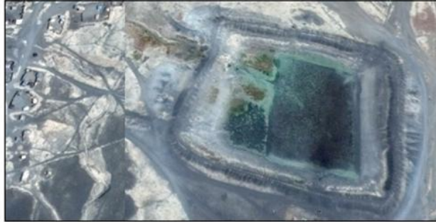
Fig. 2, Typical existing rainwater harvesting system (Hafeer), in the study area (dry season, empty).
