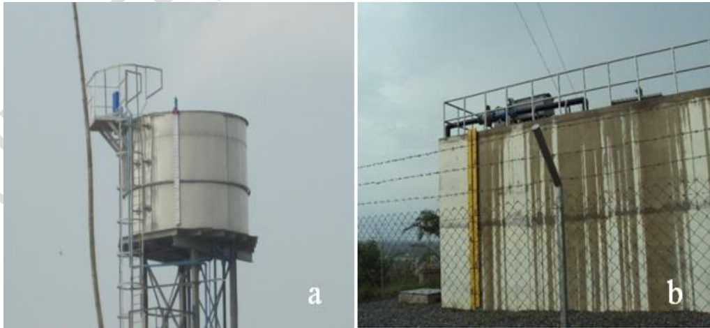
Plate 3. Service reservoirs of the AFSTWSS (a) Elevated aluminium reservoir; (b) Ground-level concrete reservoir (Source: ANMA [20])
