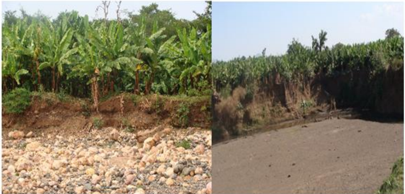
Figure 6: Siltation and Gullies formation in lower part of kulfo watershed
