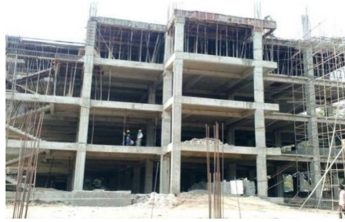
Plate 1. Typical RC frame building [7]
