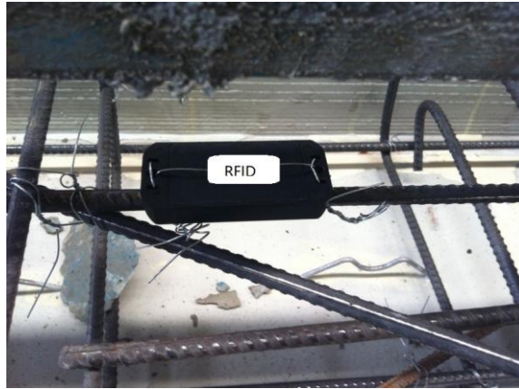
Fig 10. RFID chip is embedded in the component
