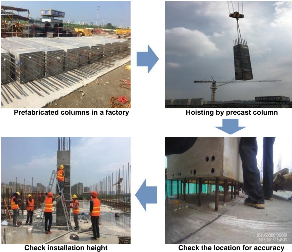
Fig 11. RFID application flow chart
