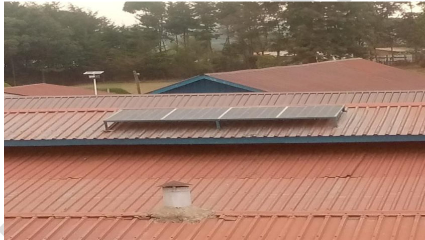
Figure 1: Photograph of the installed PV Array on the institution's social/ dining hall roof.
